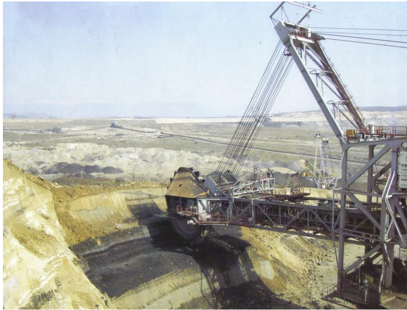
Large capacity equipment for excavation (scrapping): excavators rotor
